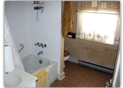
Before Full Bathroom Renovation
